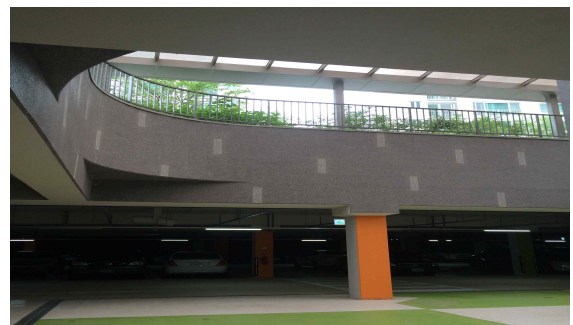
Figure 13. E apa.: Installation of sunken
