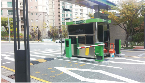
Figure 3. F apa.: Car entrance blocker
