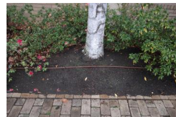
[Figure 3] Irrigation lines (Wilson Avenue)
